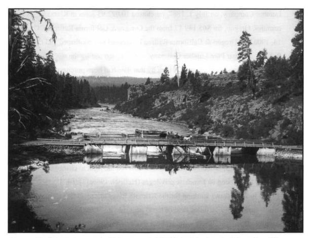
Figure 47. Splash dam west of Keno, erected 1889, to drive logs to Klamathon (Shaw Historical Library, Helfrich Collection # 860).
