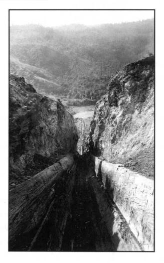
Figure 53. Planks lining Pokegama log chute (Photo courtesy of Siskiyou County Museum, Yreka, California, P03632 L Klamathon/Pokegama 19).
