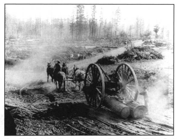
Figure 58. High wheels and horse team hauling logs (Photo courtesy of Siskiyou County Museum, Yreka, California, P03759 L T/High Wheels 1).
